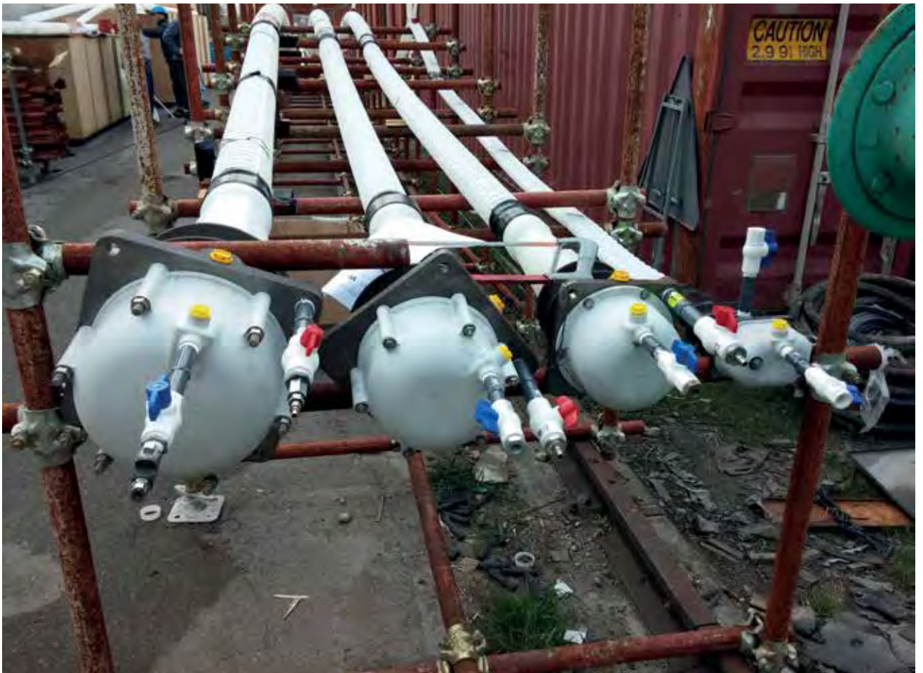
Full scale pressure tests
